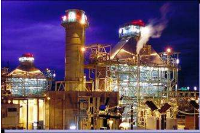
Alstom Power Sector
